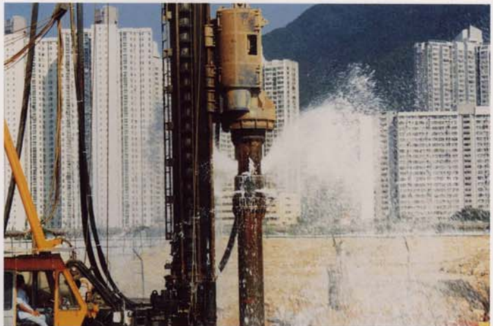
Foundation Foundational construction of buildings and bridges up to 32" (Ø800) of casing diameter.
