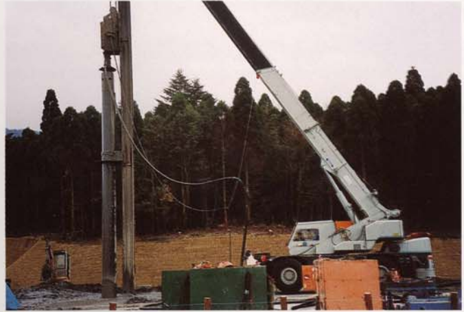
Geothermal · Oil Well Surface drilling down to 50m in depth for geothermal and oil well.
