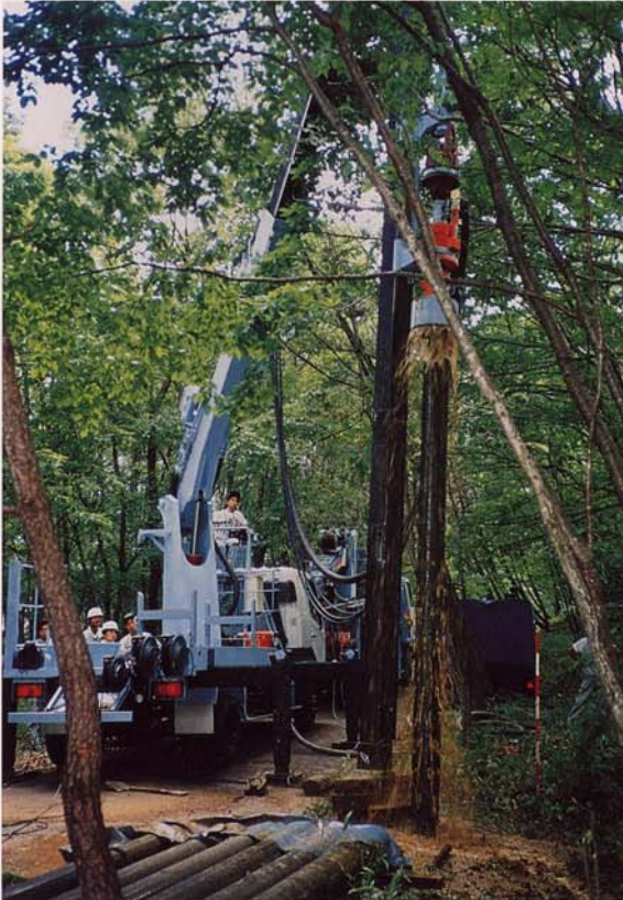
Water Well Drilling water wells down to 50 ~ 250m in depth.
